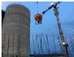
Slipform Construction
